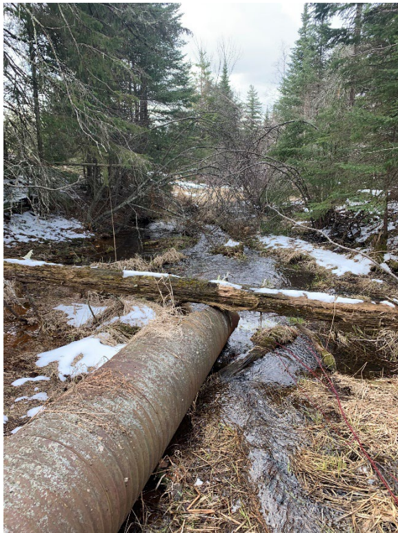
Photo 3: Outlet of Downstream Embankment
