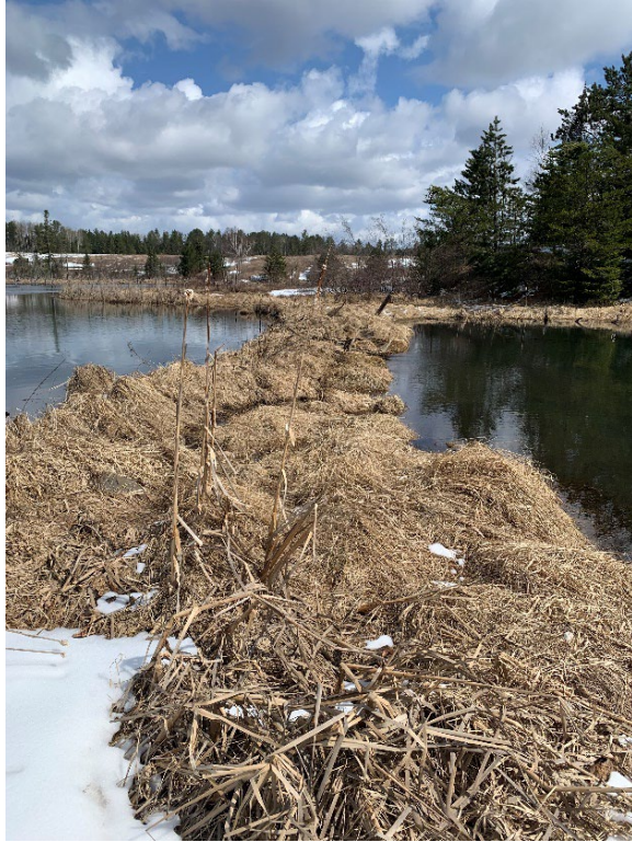
Photo 2: Embankment Looking East
