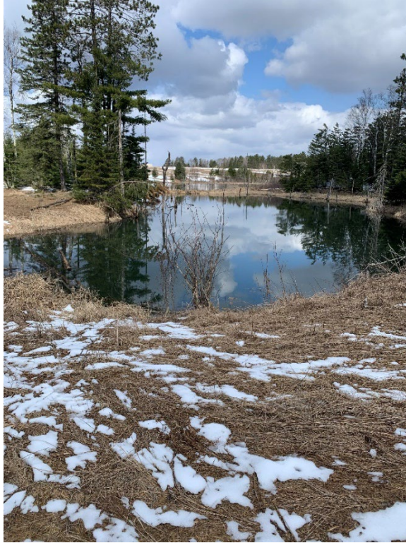
Photo 4: Downstream Impoundment looking North
